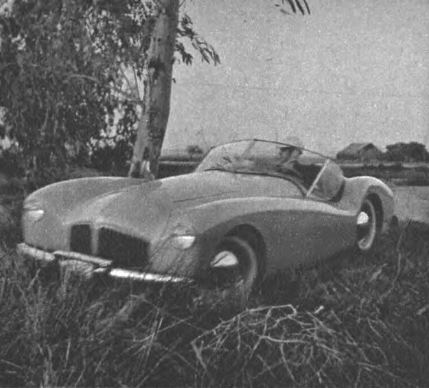
To illustrate fact that plastic body does not dent, this car sideswiped tree while going 25 miles per hour.
