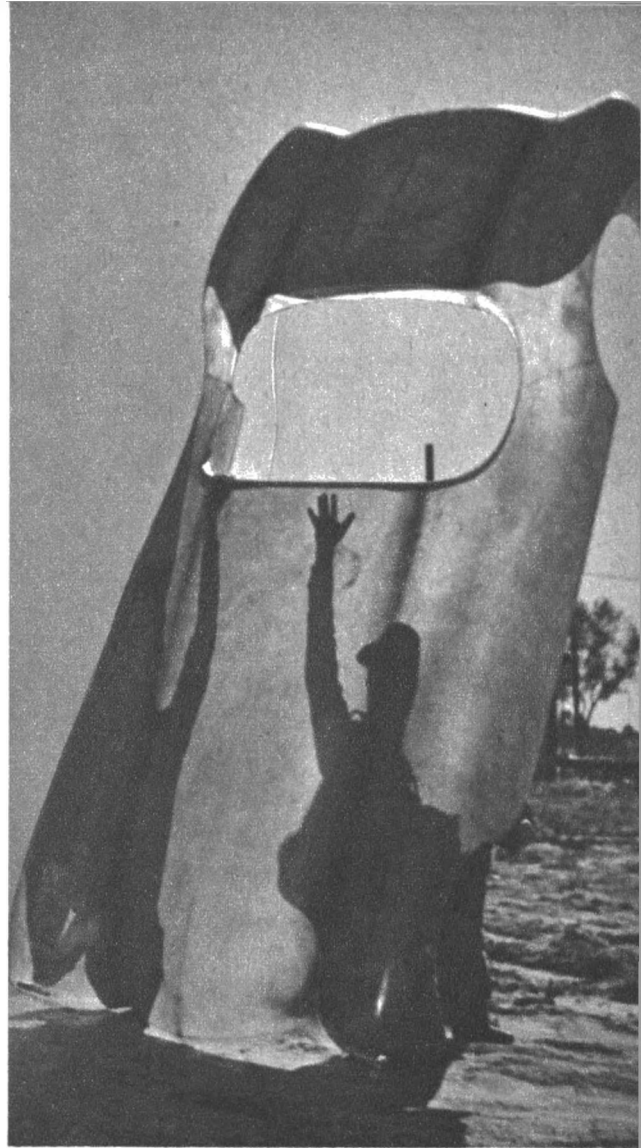
Unpainted, though finished, this translucent plastic auto body is stood high in air to demonstrate its one-piece construction and its extremely light weight of 200 lbs.
