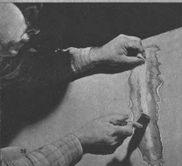
Glass fiber is laid over crack and coated with resin, then sanded and painted. Entire job took one hour.
